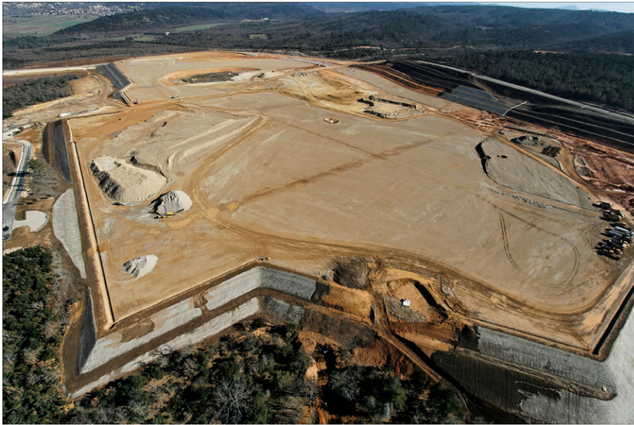
Figure 10. The levelling of the 40 ha ITER platform is now complete.
